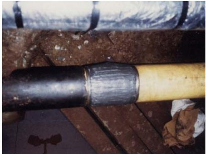
A leakage in a 154 KV P.O.F. insulation pipe was sealed using MM-metal oL-steelceramic and Hardener red working with the direct-MM-bonding method. In addition corrosion damages of the piping were removed by applying MM-metal SS-steel, liquid and Hardener yellow, liquid. Oil pressure 200 psi, diameter of the piping 300 mm, oil quality polybdenum.
