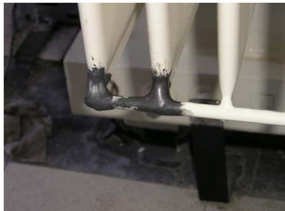
The welding at 19 places of transformers had micro cracks and blowholes, where oil exuded. First the paint has been removed with an electro drill equipped with an abrasive tool and the metal has been cleaned at the defective areas. Then MM-metal oL-steelceramic with Hardener red and afterwards Hardener yellow was applied. After checking the tightness of the repaired areas the corresponding areas have been painted over again.
