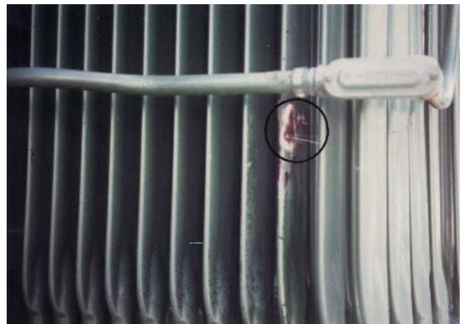
method4: Situations, where the damaged components are not subjected to vibration, or any other movements, oil leaks can be repaired by application of the PolymerMetal MM-metal oL-steelceramic alone.
