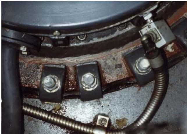
At the on-load tap changer of a large transformer oil was penetrating through cracks between the top and the on-load tap-changing equipment. The direct-MM-bonding method was used to solve this repair problem. It was carried out with MM-metal oL-steelceramic and Hardener red and afterwards Hardener yellow.
