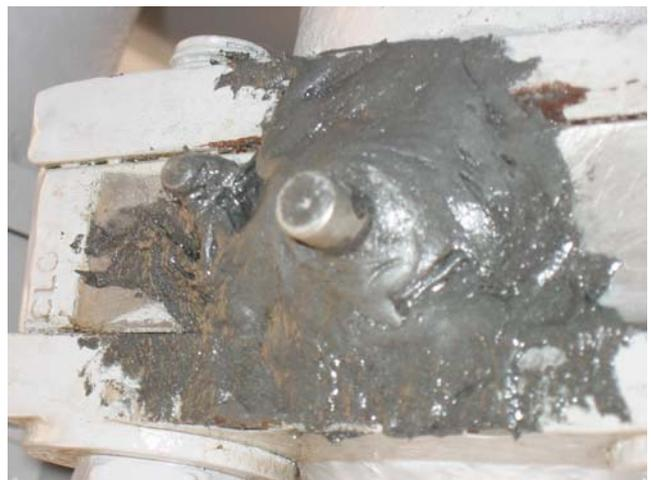
A damaged power transformer located in a steel plant has been repaired by using MM-metal oL-steelceramic and Hardener yellow.
