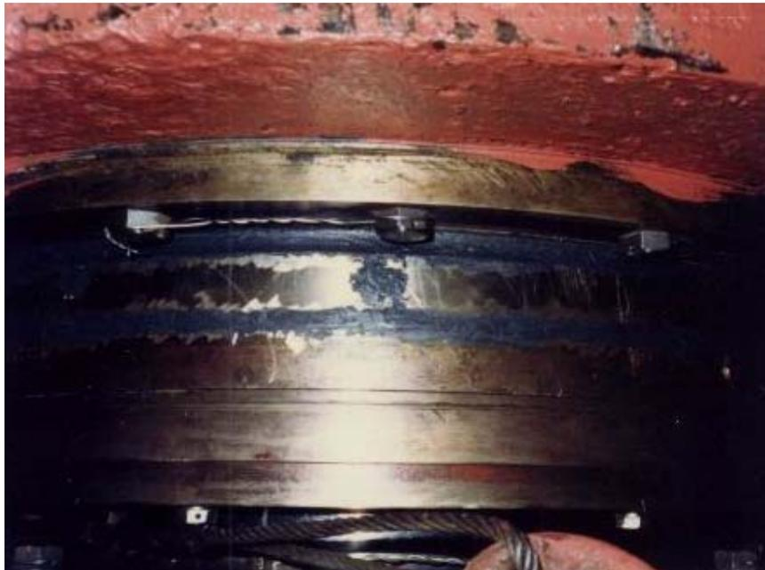
Repair of a leaking simplex compact packing. The repair was difficult due to oil pouring out of the repair site. Therefore it was decided to use the direct-MM-bonding method by applying the PolymerMetall directly on the greasy surface. Here MM-metal oL-steelceramic with Hardener red was chosen.
